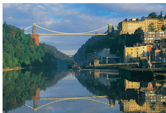
Clifton Suspension Bridge
